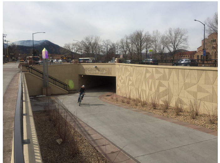
Figure 30: Boulder's 80th Underpass at Baseline between Broadway and US 36 (Source: City of Boulder)
