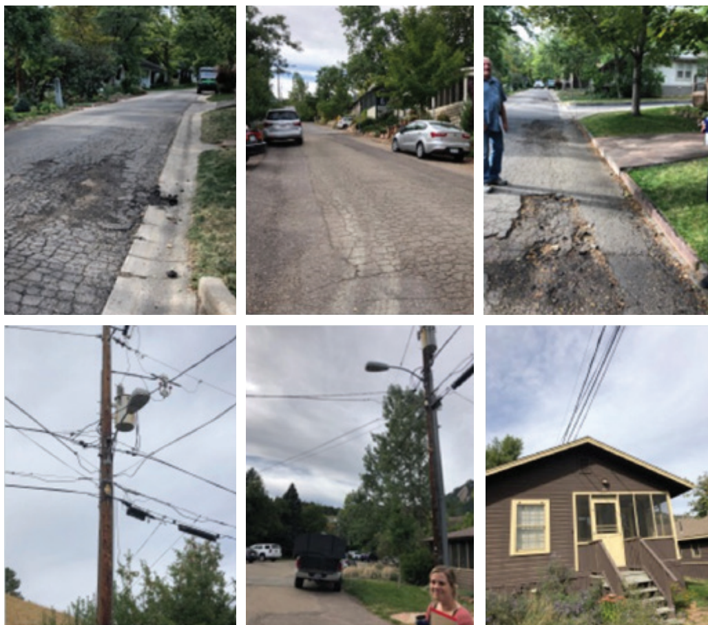
Figure 19 (top row): The increasing temperature profile at Chautauqua is causing roads to break down as asphalt surfaces are not design for the environmental conditions at the site.
