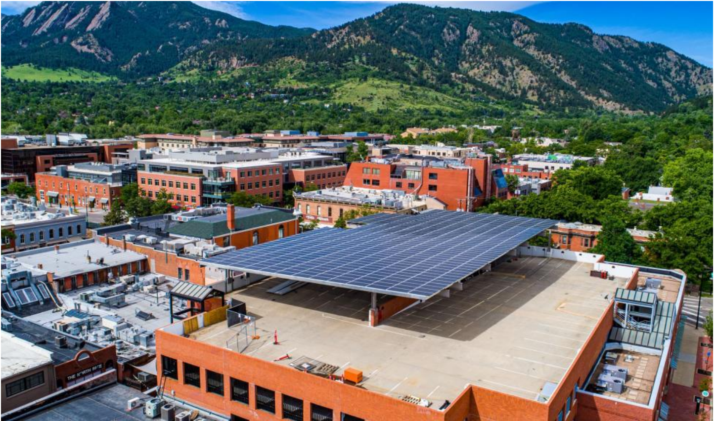
Figure 9. More than 2 MW of solar power is generating renewable energy and reducing operation costs at 19 City of Boulder facilities
