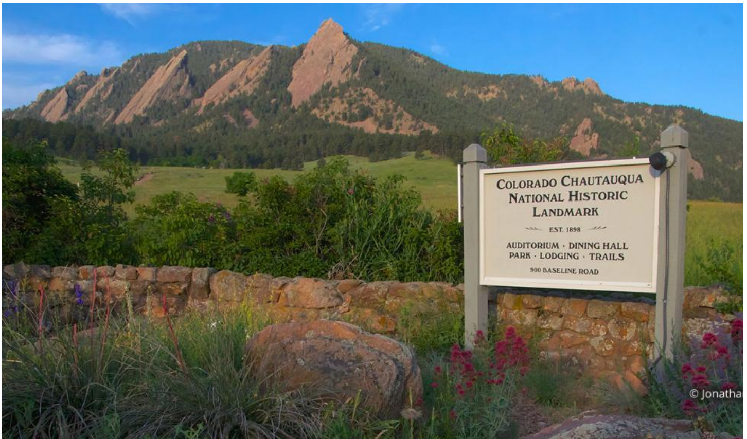
Figure 10. The Chautauqua Sustainability & Resilience Strategy will increase reliability and reduce the risk of wildfire
