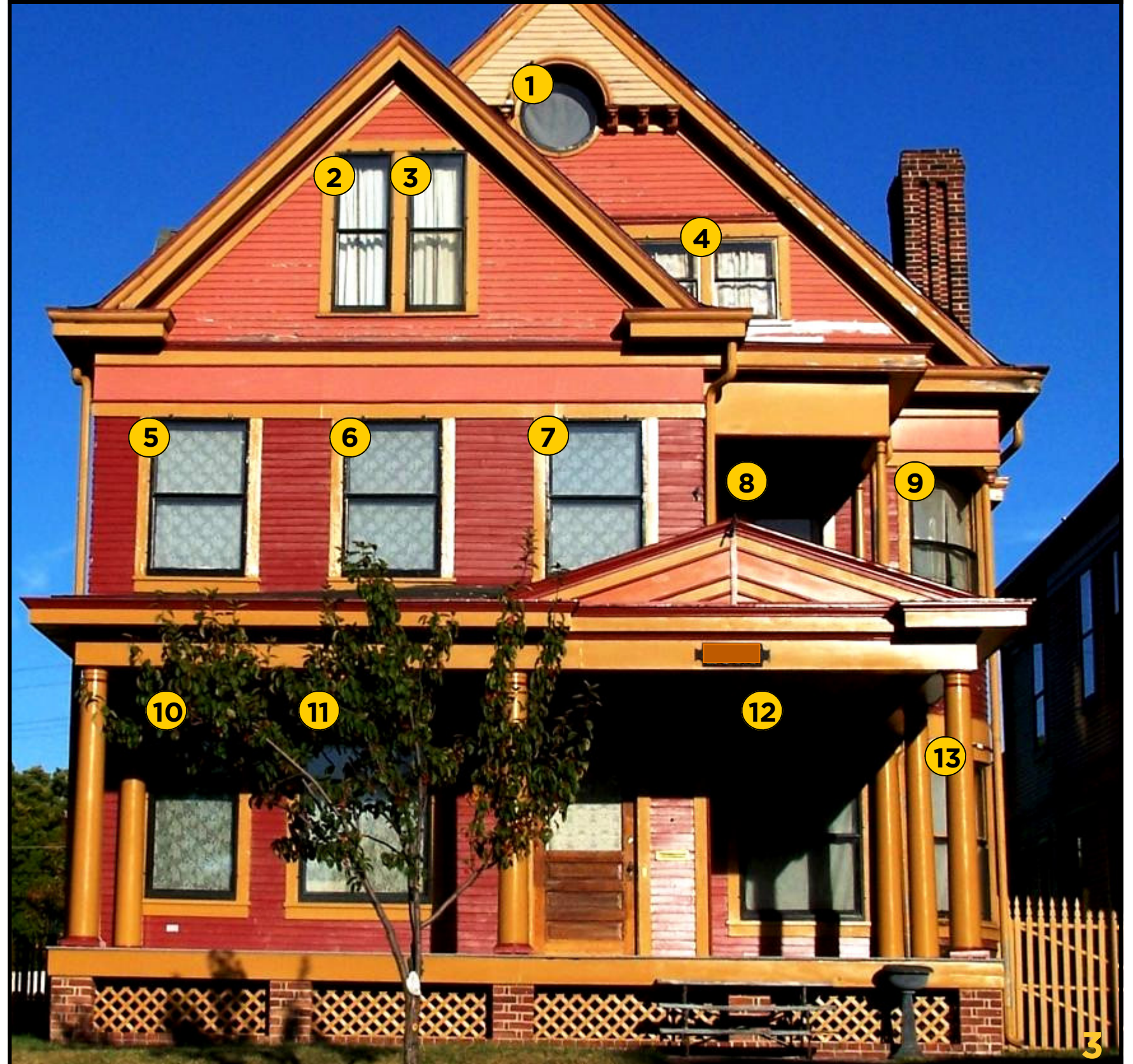
1890s Queen Anne style house Original one-over-one double-hung sash windows with storm windows
