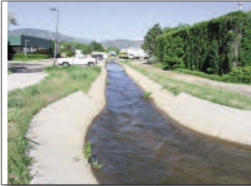
A path planned along the North Boulder Farmer's Ditch will connect the Transit Village to Twenty Ninth Street.
