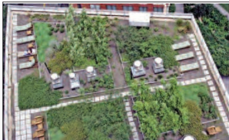
Green roofs are one of the stormwater best management practices that will be encouraged.
