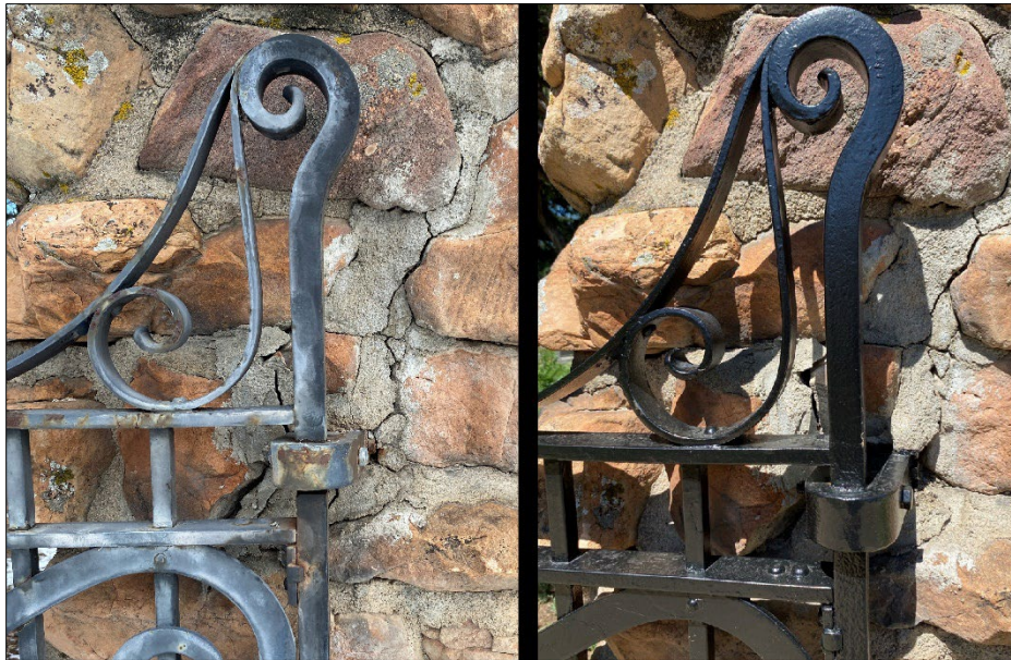
Repaint Fence: Before and After
