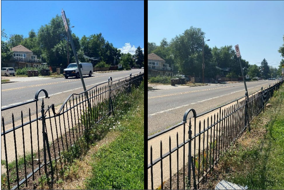
Fence and Gate Repairs: Before and After
