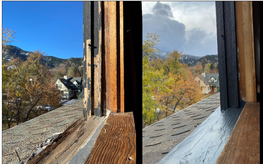
Window Sill Repair – Before and After
