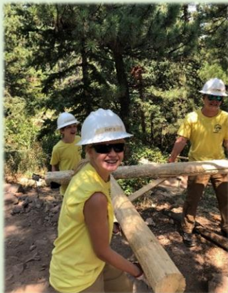
INSTALLING BUCK AND RAIL FENCE TO ENCOURAGE TRAIL USERS TO STAY ON THE TRAIL AND RESTORE TRAMPLED AREA.
