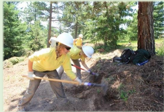
REMOVING EXCAVATED MATERIAL FROM TREAD ROUGH CUT (ABOVE), DEFINING THE BACKSLOPE AND MAKING TOP CUT OF NEW TREAD (BELOW), & DEFINING INSIDE HINGE AND BACKSLOPE (LEFT).
