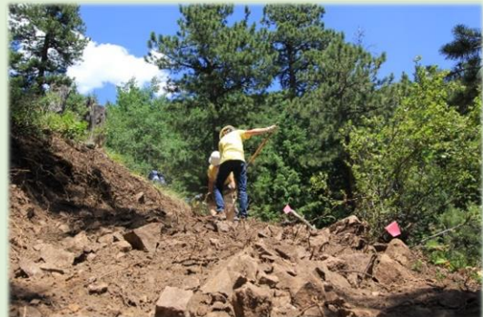
REMOVING EXCAVATED MATERIAL FROM TREAD ROUGH CUT (ABOVE), DEFINING THE BACKSLOPE AND MAKING TOP CUT OF NEW TREAD (BELOW), & DEFINING INSIDE HINGE AND BACKSLOPE (LEFT).
