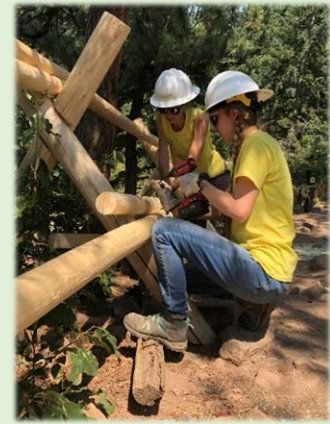
INSTALLING BUCK AND RAIL FENCE TO ENCOURAGE TRAIL USERS TO STAY ON THE TRAIL AND RESTORE TRAMPLED AREA.
