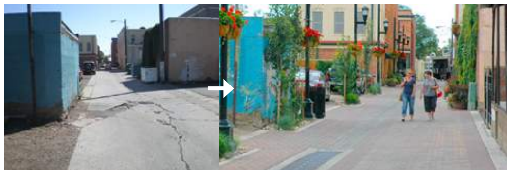
Provide a uniform, well drained surface with inverted crown drainage and no more than 2% cross-slopes
