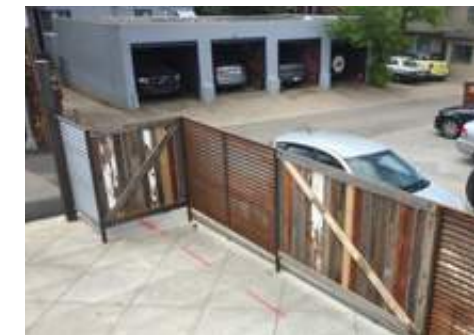
Build on materials in 'The Hill'
