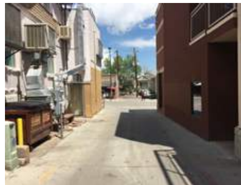
Inconsistent private property upgrades
