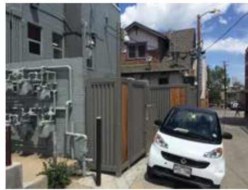
Trash enclosures and private property improvements in progress
