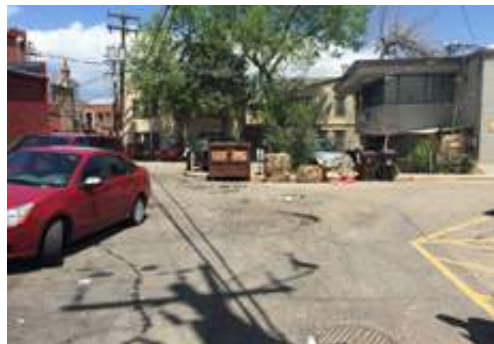
Lack of definition between alley R.O.W. and parking
