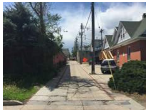
Overhead lines dominate sight lines, no defined entry
