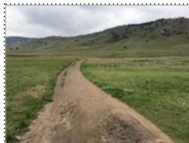
Foothills South Trail after 2013 flood, photo: OSMP
