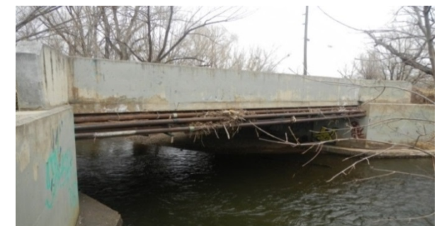
Photo 22: Old Valmont trail bridge (Reach 7)
