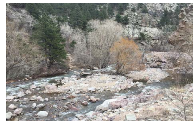
Photo 33: Deposition in Boulder Canyon (Reach 10)
