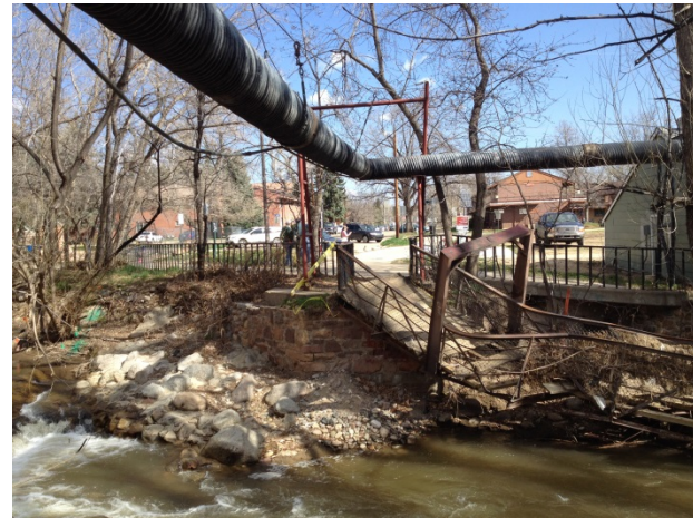
Photo 27: 19th Street Pedestrian Bridge (Reach 9)
