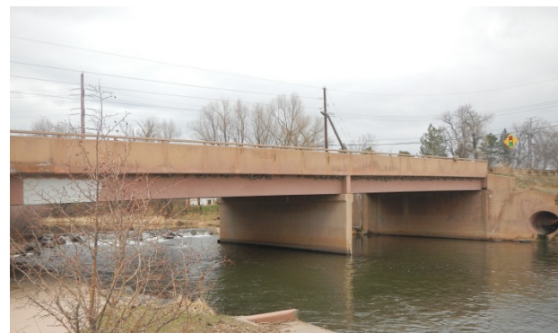
Photo 17: 75 th Street Bridge (Reach 6)
