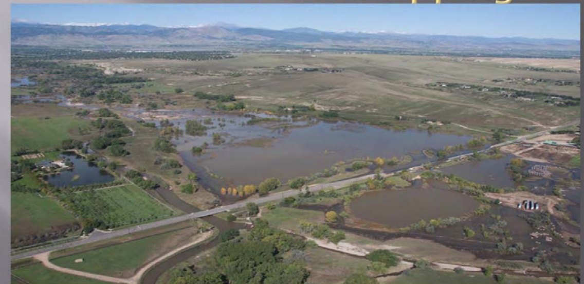
95 th Street Overtopping - David Mallory, UDFCD 2013
