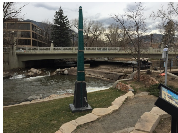
Photo 29: Downstream Broadway Bridge (Reach 9)
