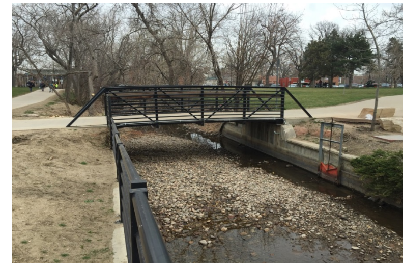
Photo 9.2 – Boulder Slough Diversion at Broadway
