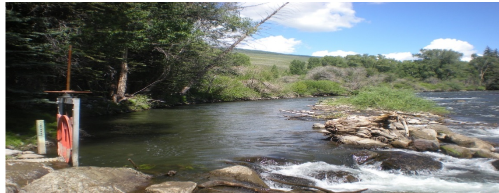
Photo 9.1 - Example of diversion structure and fish passage channel (ERC, East River)
