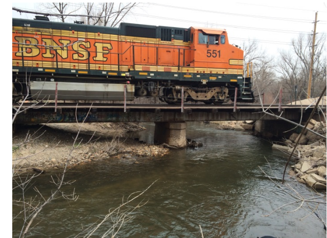
Photo 26: BNSF Railroad Bridge (Reach 8)
