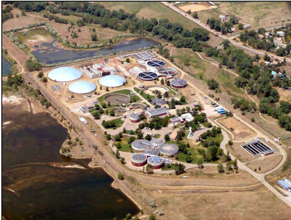
Figure 2. City of Boulder 75th Street Wastewater Treatment Plant
