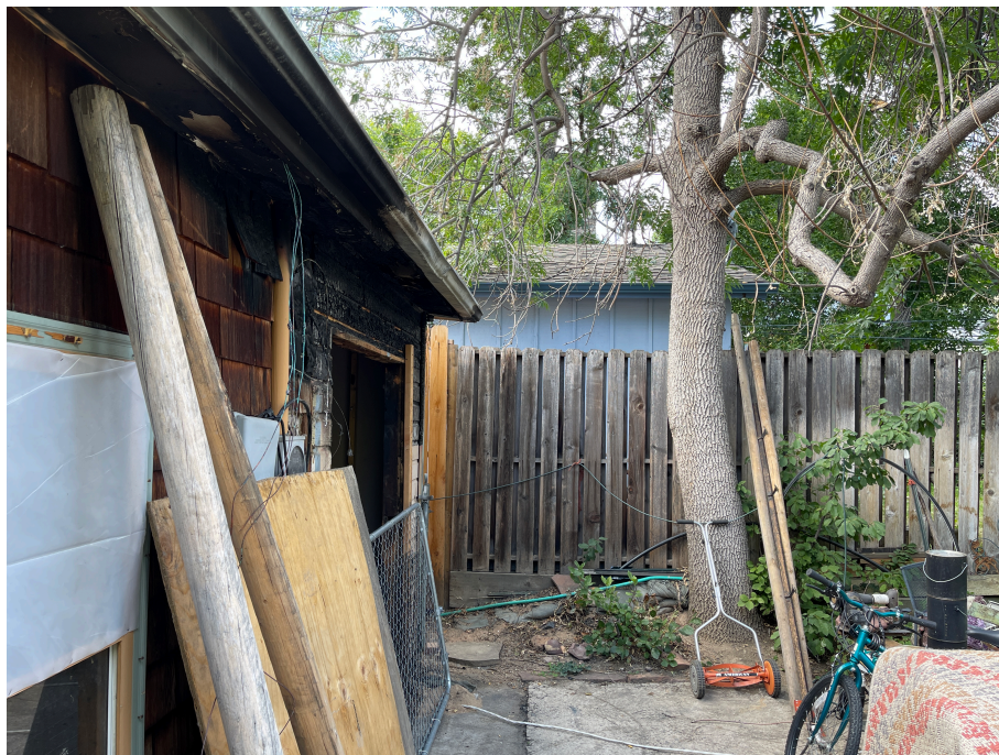
View along North side of existing structure to the West
