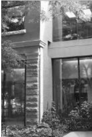
A new addition set back from the block face
