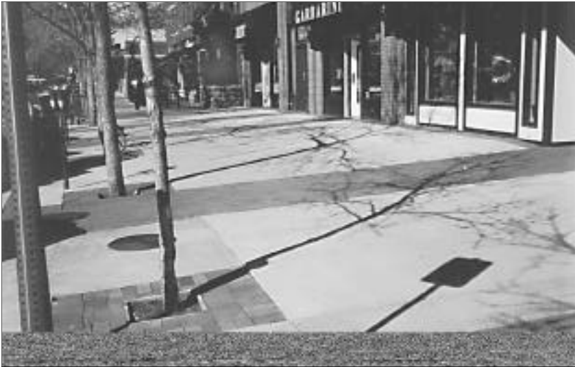
Brick paving used to highlight entrances.
