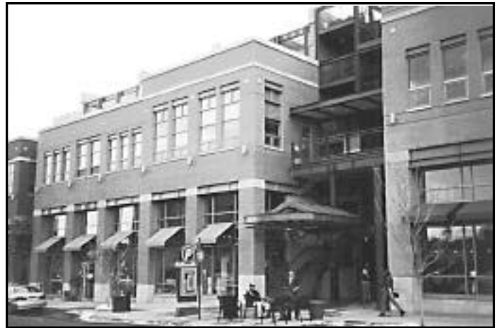
Design with traditional commercial features, this parking facility has retail/commercials spaces along the street
