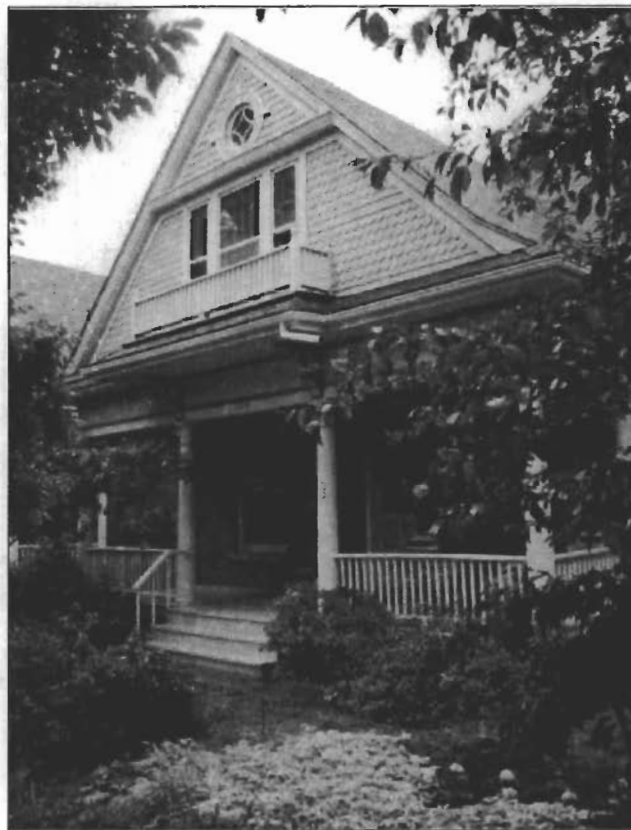
Use traditional materials, such as those above, to enhance the visual character of the site.
