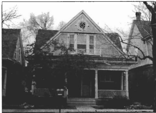
Shingled gables, prominent porches and decorative detailing are all characteristic of the Queen Anne style.
