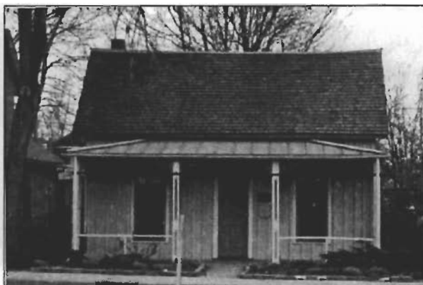
This house at 1733 Canyon Street is an excellent example of a vernacular wood frame house.
