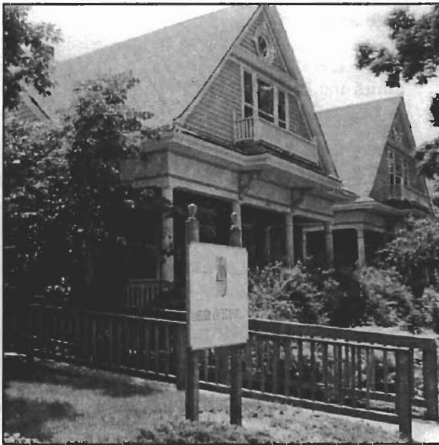
G.3: Alterations to historic properties that are designed to improve access for persons with disabilities should create minimal negative effect on the historic character or materials.
