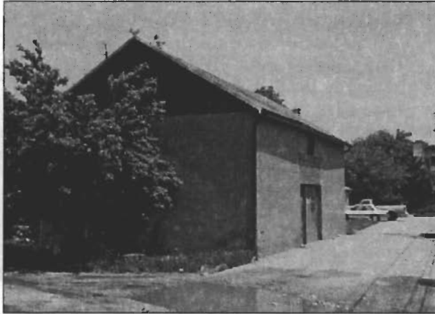
Historic accessory structures, such as the one above, help define the alley edge.
