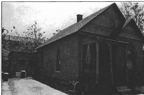
This masonry house, similar to many seen throughout Boulder, was constructed in the vernacular—meaning that it was not based on a high style, but rather built as a modest, functional dwelling.
