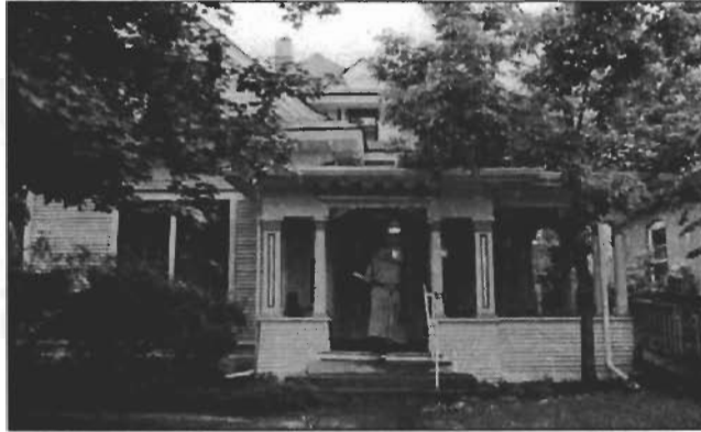
With its hipped roof, central dormer, flared eaves and doric columns, this house at 1628 Walnut represents a typical Classic Cottage.
