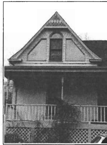
These trapezoidal windows do not relate to the type or proportion of the existing double hung windows in this house.
