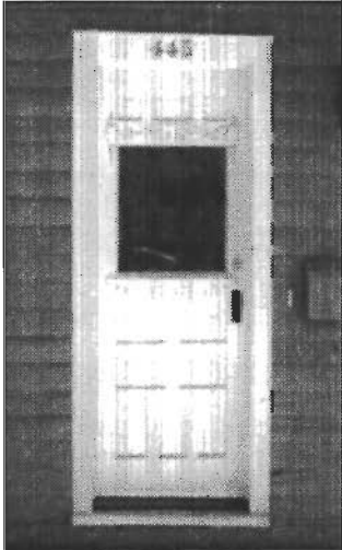
This paneled wood door features original ornamentation.
