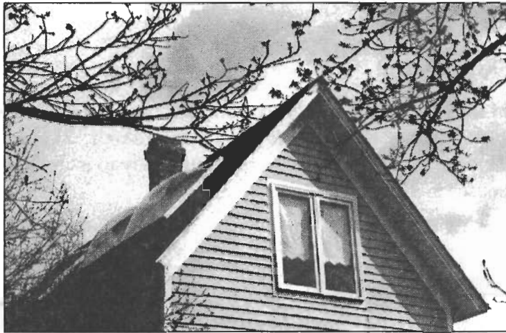
These “bubble” skylights detract from the character of this house.
