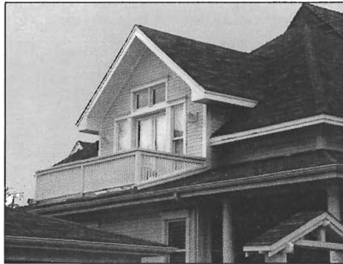
This deck is appropriately incorporated into the roof.
