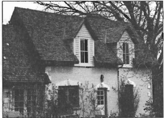
These new dormers add usable space to the second floor while maintaining the integrity of this house.
