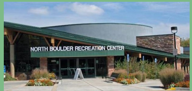
North Boulder Recreation Center – Targeted Improvements for HVAC equipment and in the building, envelope will be recommended.
