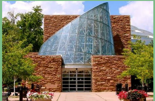
Main Library – Recent building controls upgrade.
