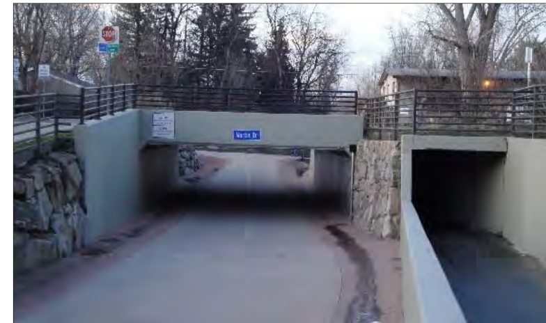
Culvert R2-8: Martin Drive
