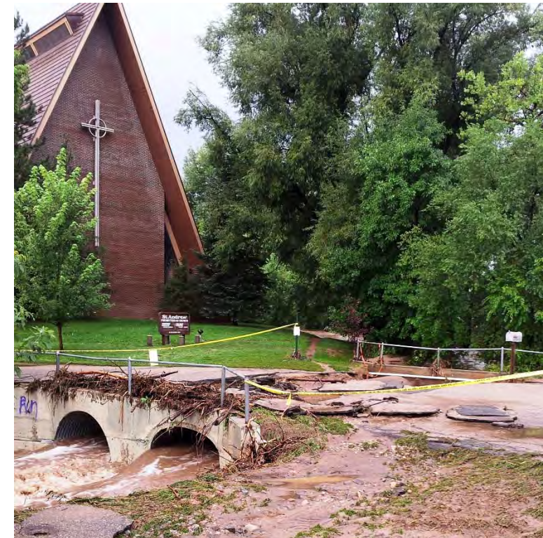
Culvert R3-3: Saint Andrew Church Driveway
