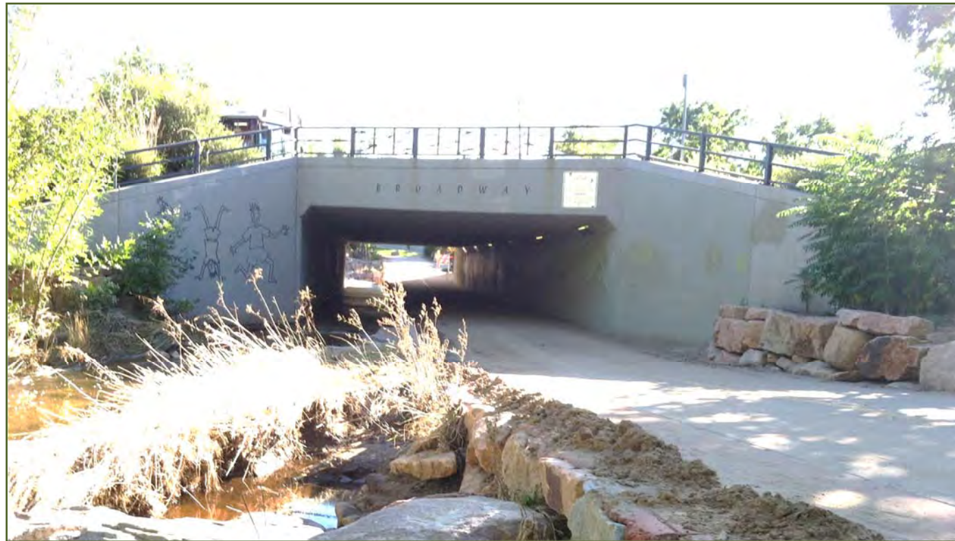
Culvert R2-7: Broadway Underpass
