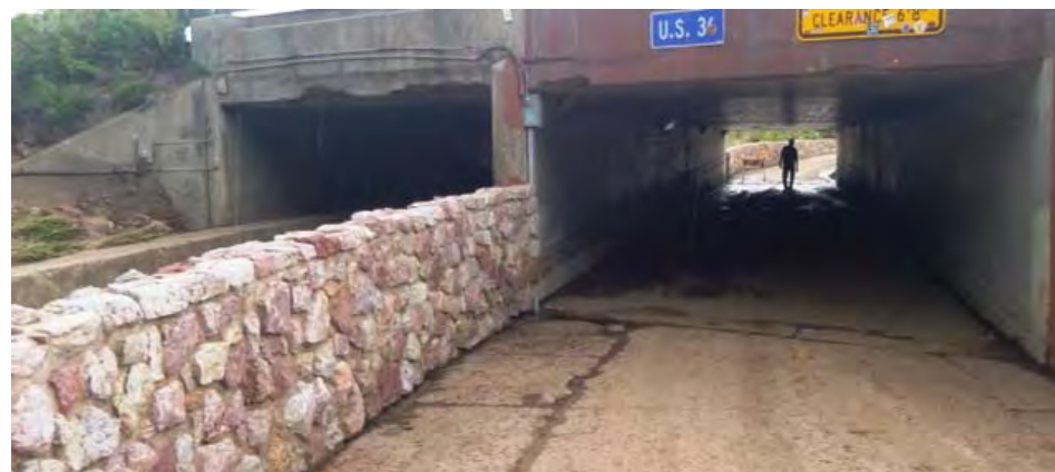
Culvert R3-2: Underpass at US 36
