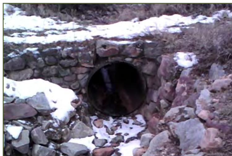
Culvert R1-2: Ithaca Drive Steel Pipe
