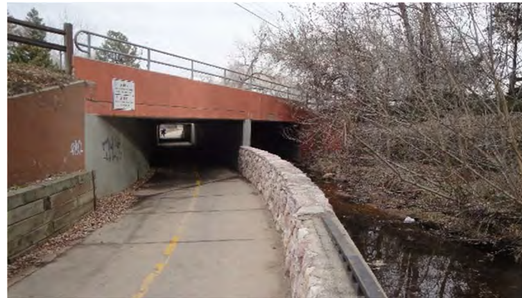
Culvert R3-4: Underpass at Baseline Road
