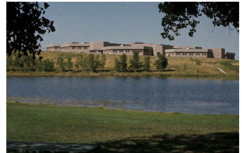
FAIRVIEW HIGH SCHOOL In 1971, modernist architect Hobart Wagener designed Fairview High School, Boulder's second high school.
