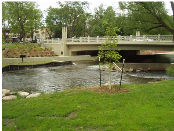
Broadway Bridge at Boulder Creek
