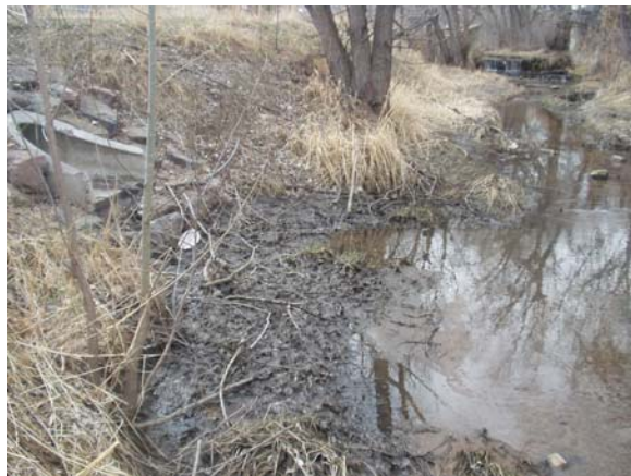
Example of Storm Sewer Discharge into an Irrigation Ditch
