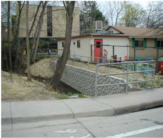
Day Care Center After Flood Mitigation Improvements
