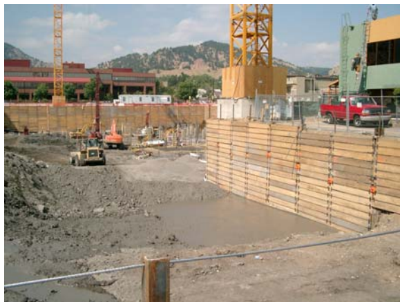
Construction Dewatering at 9 th & Canyon
