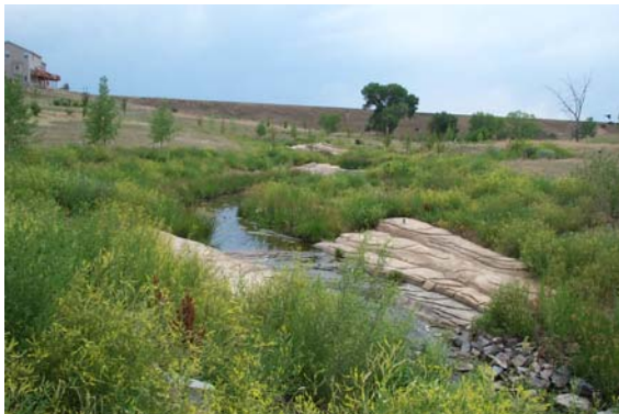
“Non-structural” Type Drainageway Constructed in the 1990s
