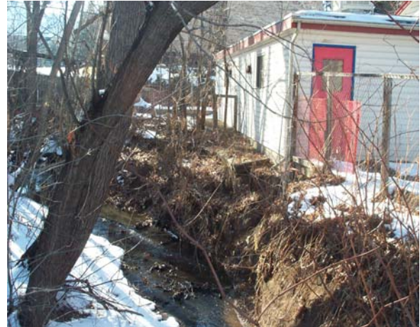
Day Care Center Exposed to Flood Hazard Risk
