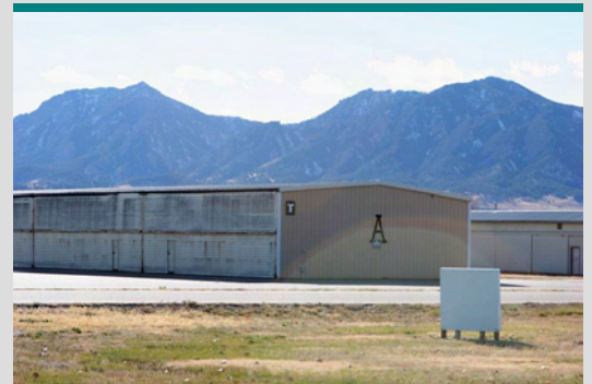
Many airport buildings are 30+ years old
