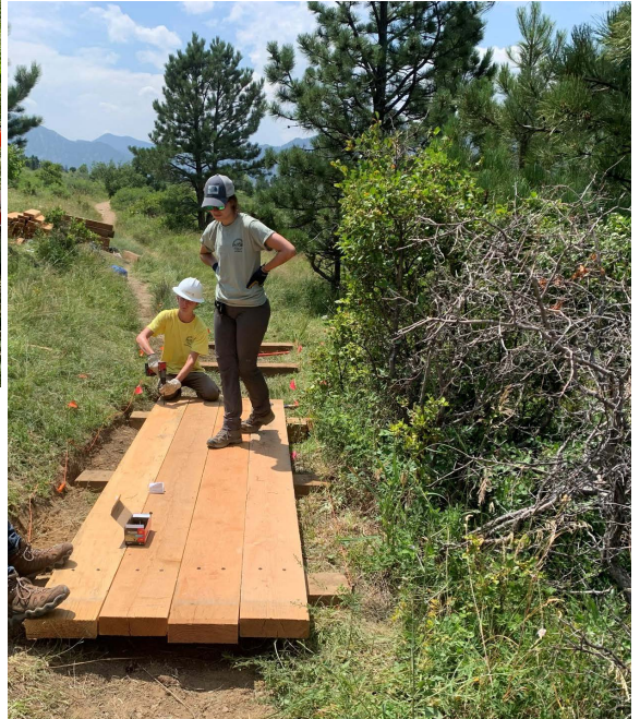
Drilling planks onto the sills to build the walking surface
