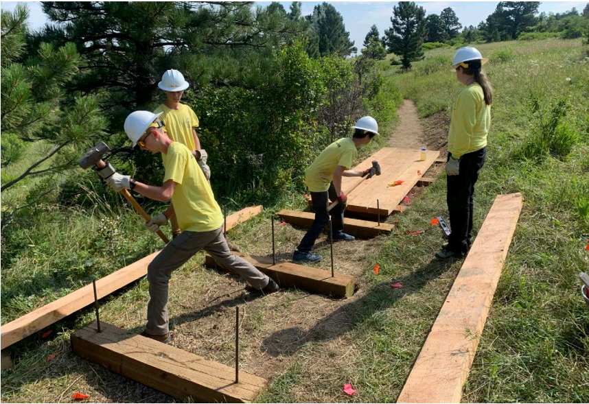
Setting sills in the ground by hammering in rebar
