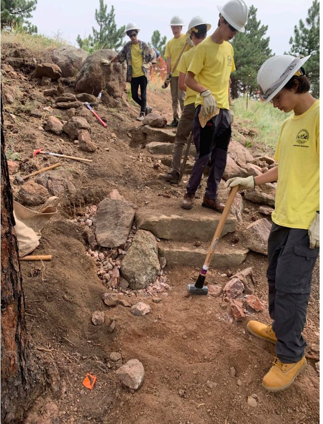
Building rock steps on the Anemone trail re-route
