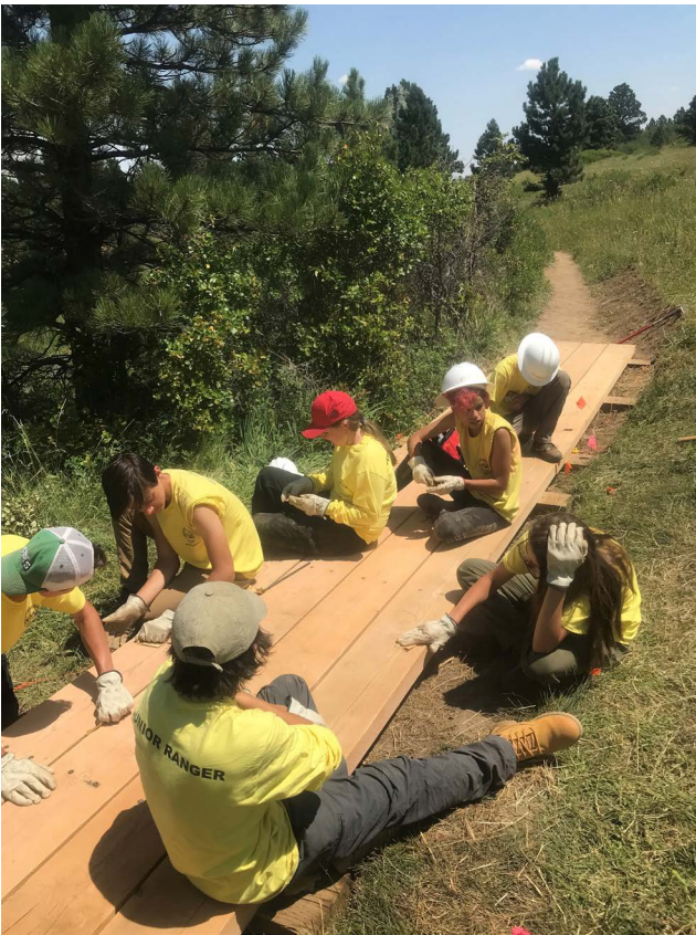
All of crew 5 joins in to sand down the wooden planks
