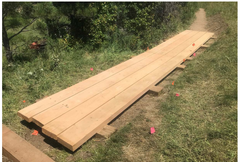
Finished! Now hikers can use the puncheon instead of walking in the mud on Marshall Mesa trail.
