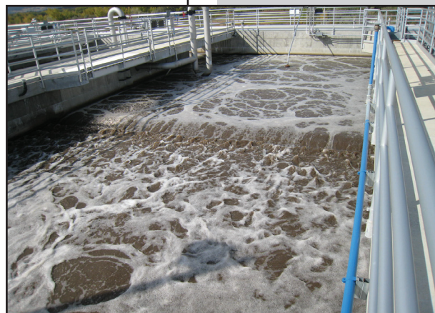
A project to replace the existing chlorine disinfection system with UV is underway at the Wastewater Treatment Plant.
