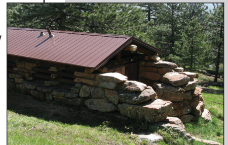
Completed repairs to the 1935 CCC Halfway House
