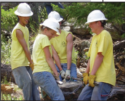
The OSMP Junior Rangers program assists in trail construction and restoration.
