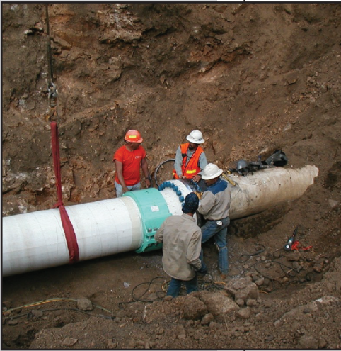
Funding for re-inspection of the Lakewood Pipeline are scheduled in 2014.
