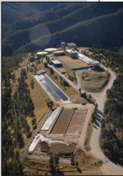
Betasso Water Treatment Plant Improvements are scheduled for 2016
