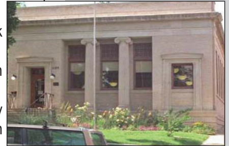
Continued exterior repairs at the Carnegie Branch Library
