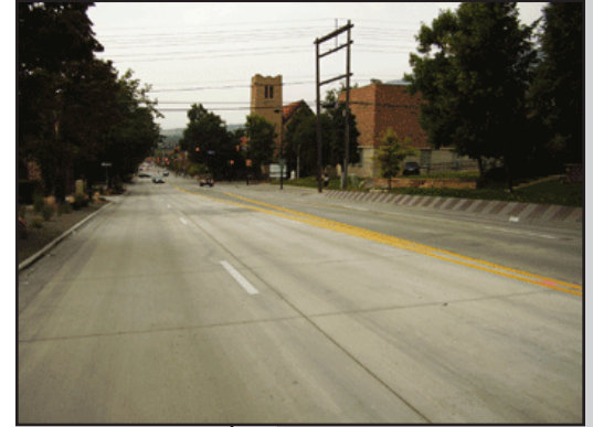
The first completed segment of the Broadway - Pine to Iris project.
