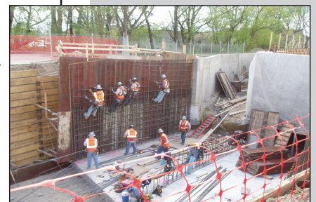
Completed construction of Elmer's Twomile Greenway Project
