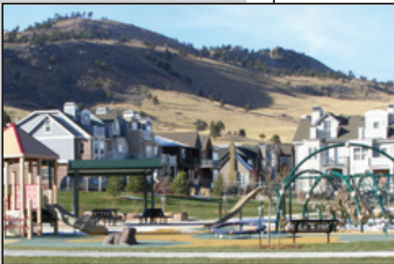
Completed Dakota Ridge Park
