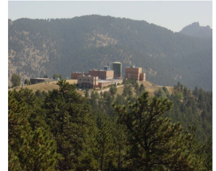
Betasso Water Treatment Facility.
