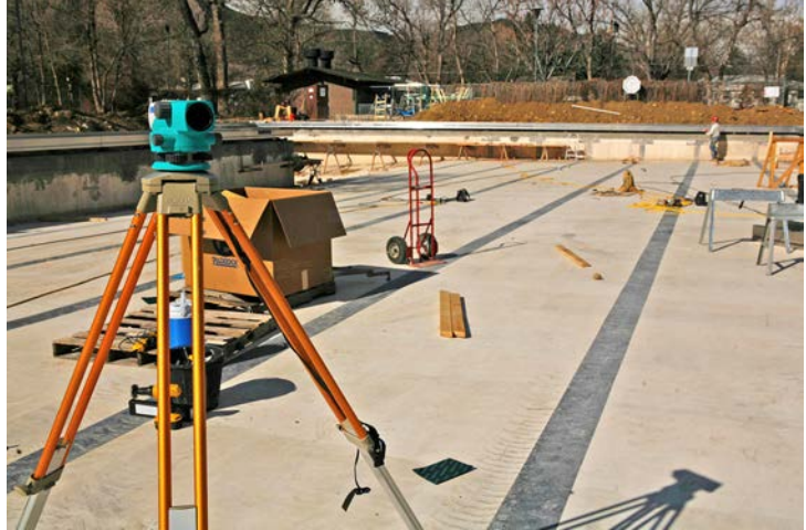
Improvements being made to Scott Carpenter Pool
