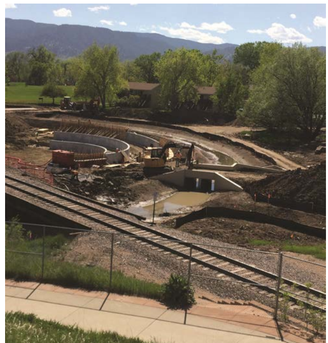
Wonderland Creek Flood Mitigation
