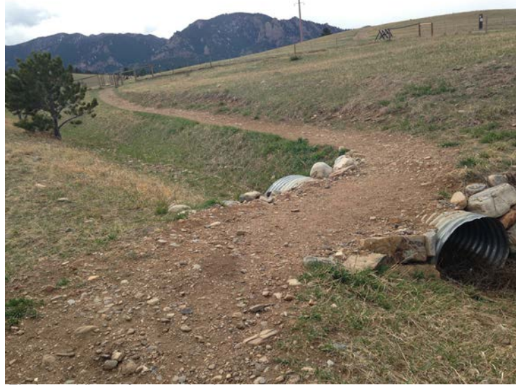
Flatirons Vista after repaired culvert
