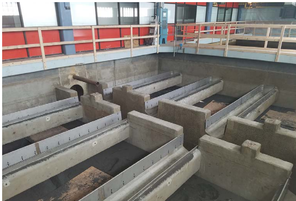
Improvements being made at Betasso (WTP)
